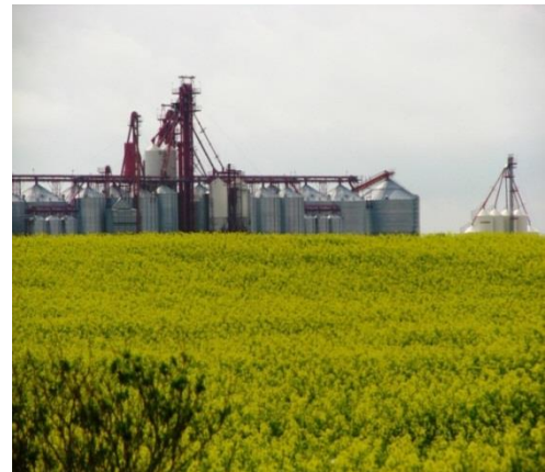
Grain Elevators, Nokomis Area
