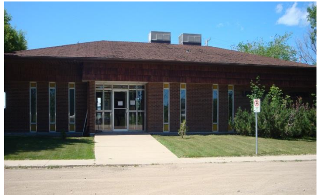
Health Centre, Town of LeRoy
